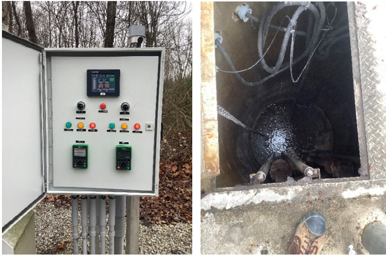
Figure 1-7 Blanches East Lift Station
