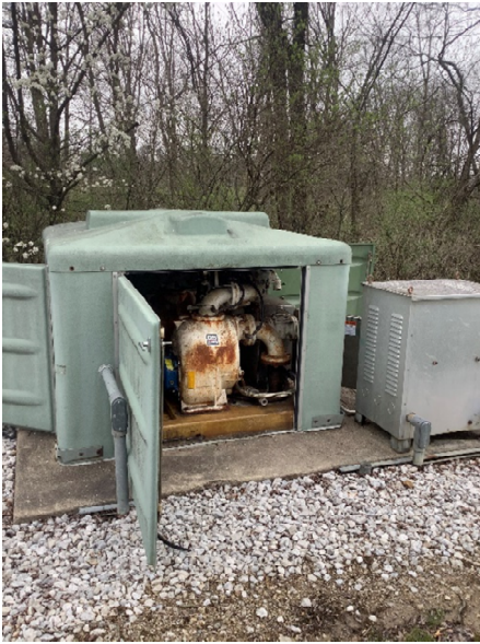
Figure 1-28 Mink North Lift Station
